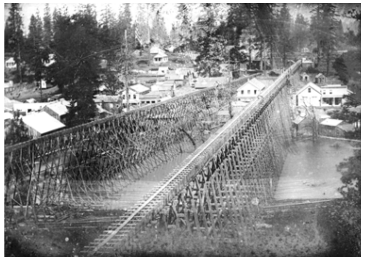
Wooden flumes carry water for hydraulic mining through North San Juan c.1870 Collection of the Searls Historical Library
